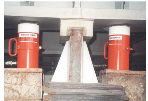
C10010C used in this lift application.
