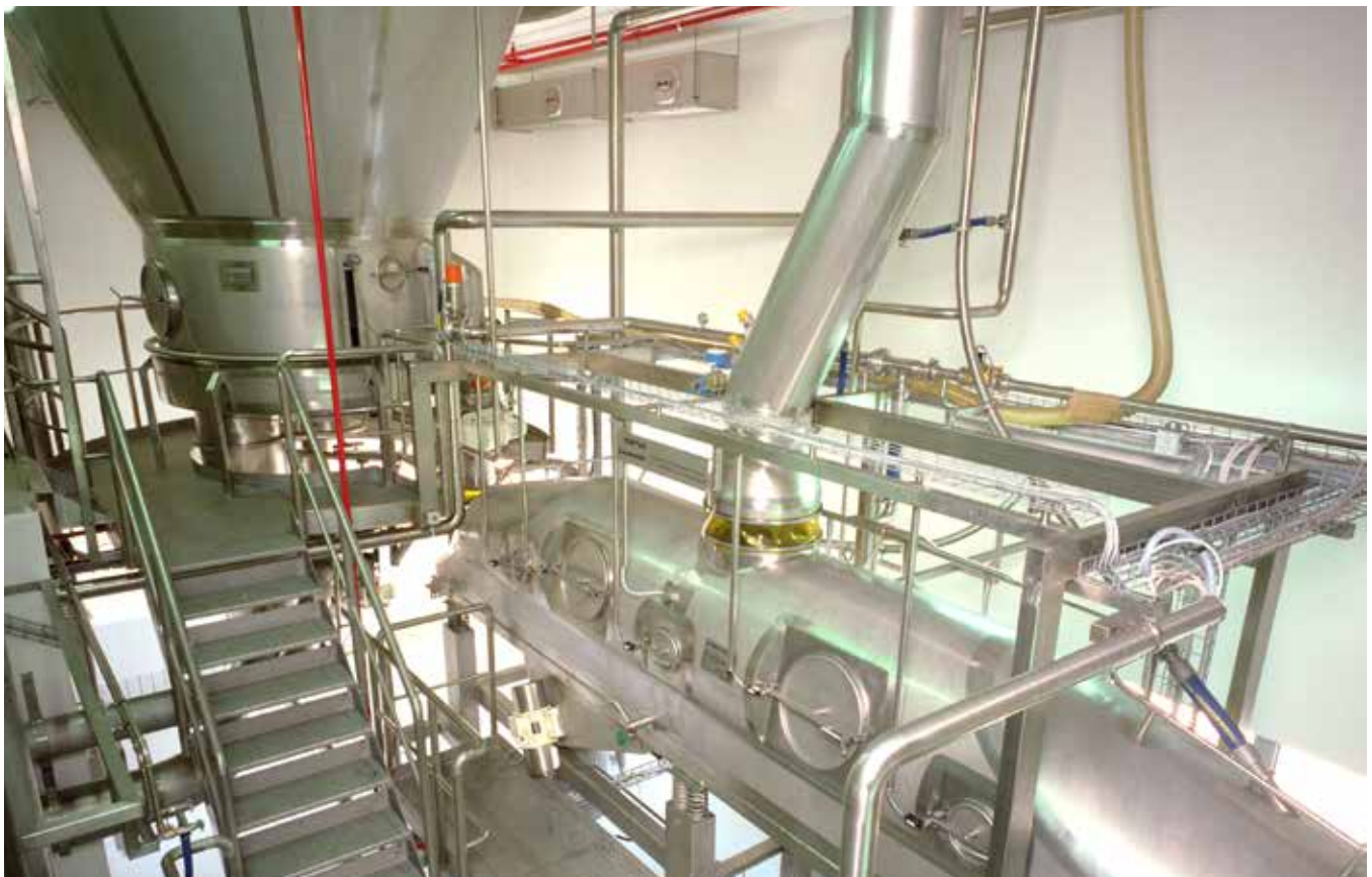
An Anhydro fluid bed in combination with a spray drying plant
