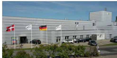
The SPX Flow Innovation Centre, Copenhagen
