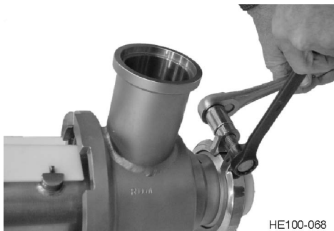
Figure 46 - Installation of Hinged Clamp
