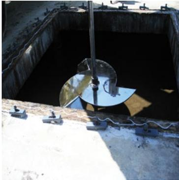
The Clean Edge impeller pictured left remains free of fibrous debris while delivering performance equal to a hydrofoil impeller.
