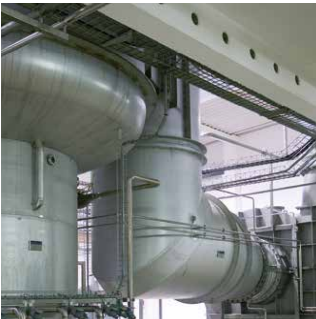
Vapor duct of MVR evaporator
