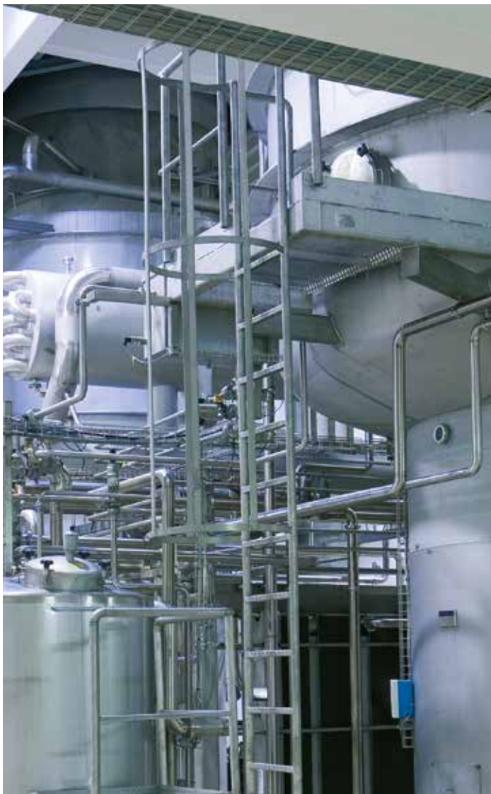
Bottom part of MVR evaporator
